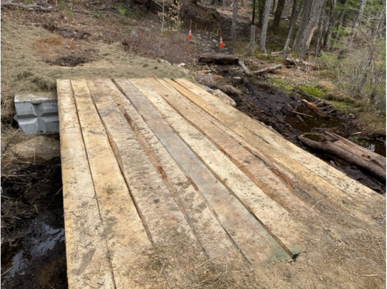
New bridge replacing an aging and deteriorated bridge, April 2023
