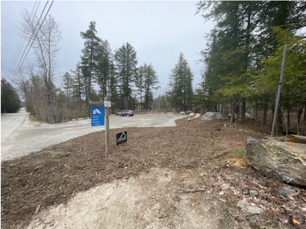
Parking lot construction (not yet complete), April 2023
